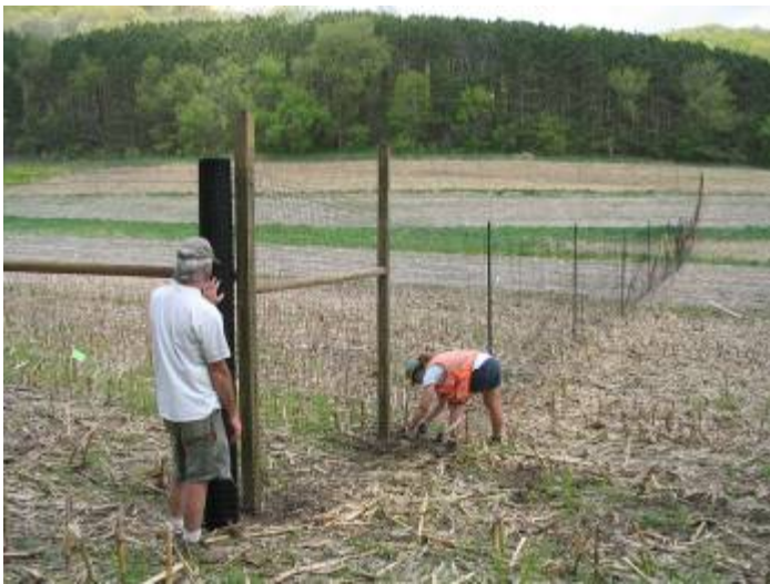
Tree Improvement crew installing deer fence in Crawford County.
