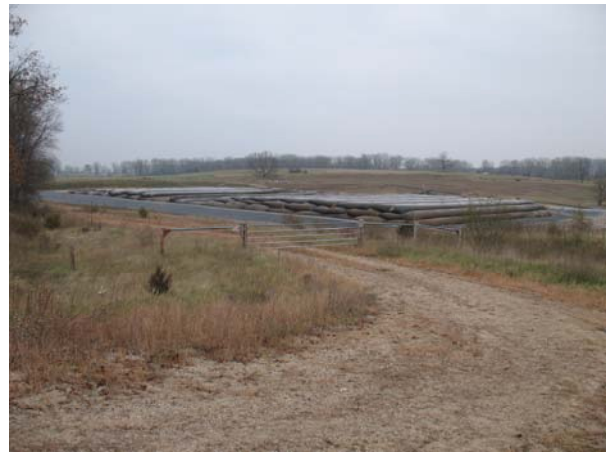
Photos of the laydown area at the Badger Army Ammunition Plant. Sediment from Gruber's Grove Bay was pumped into these geotubes, where it will remain. The laydown area is lined and will be capped in spring 2007. Photos by Hank Kuehling.
