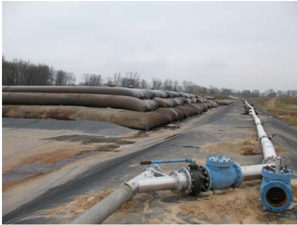
Photos of the laydown area at the Badger Army Ammunition Plant. Sediment from Gruber's Grove Bay was pumped into these geotubes, where it will remain. The laydown area is lined and will be capped in spring 2007. Photos by Hank Kuehling.
